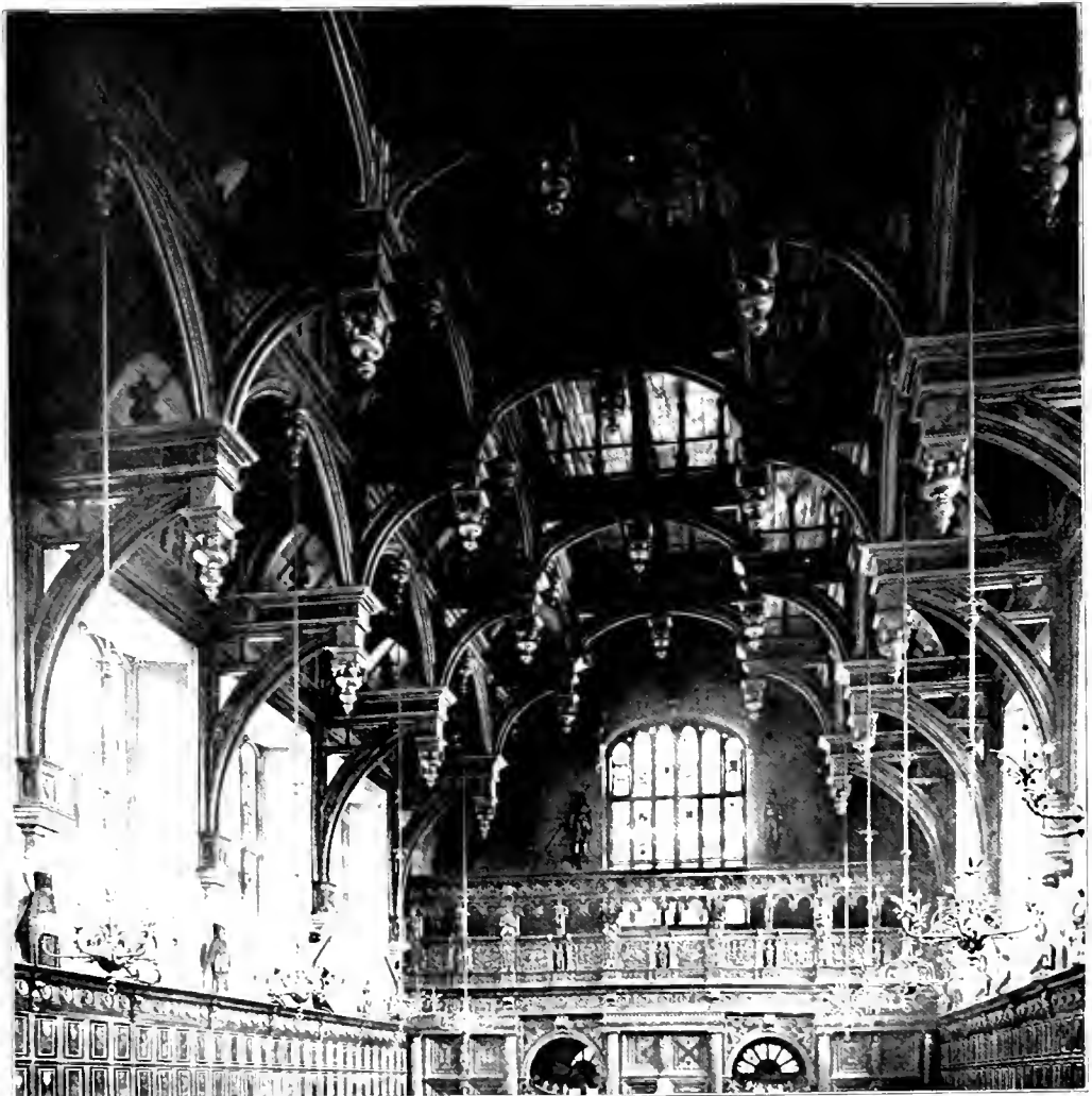
OPEN TIMBER ROOF, MIDDLE TEMPLE HALL, LONDON
